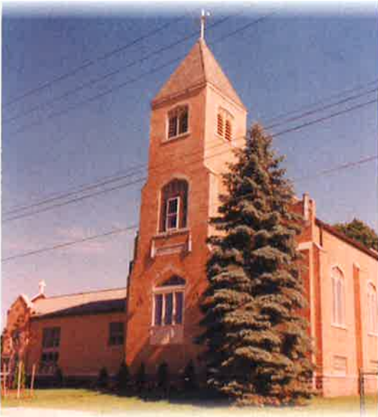
Oakfield Site 56 Maple Ave., Oakfield
